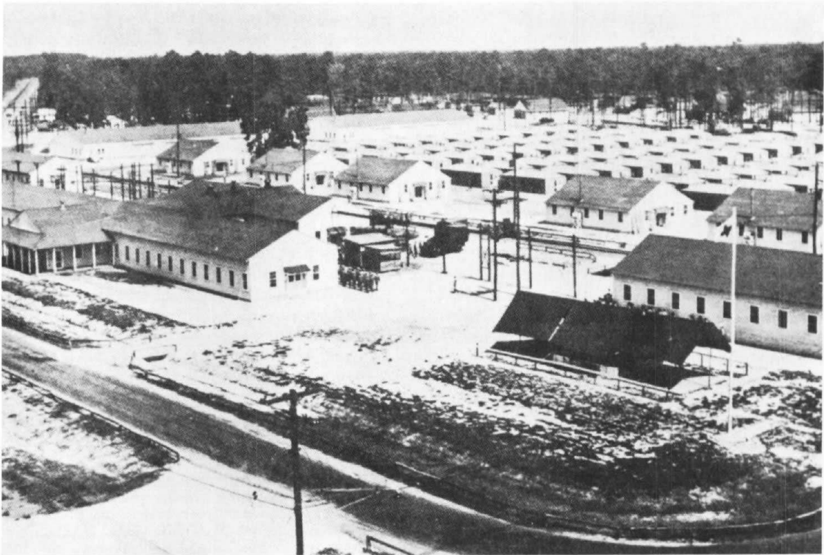
Montford Point Camp as it appeared in 1943. In the left center is the mess hall; in right center are the "little green huts" of boot camp. (Photo from Montford Point Pictorial).
